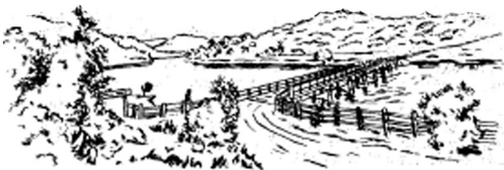
Woronora bridge as seen in 1920
