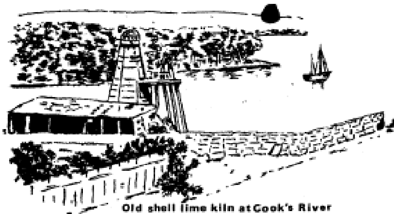
Old shell lime kiln at Cook's River
