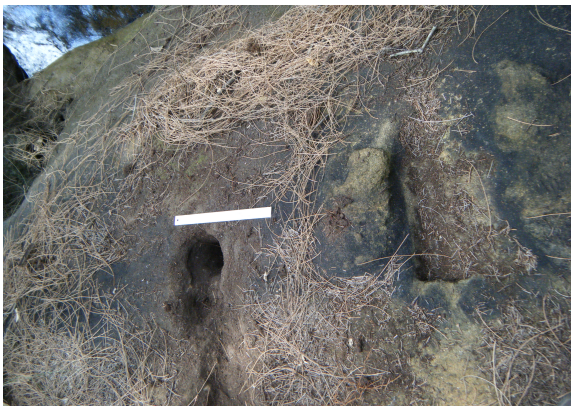
Photo 4: Cutting and large hole in a rock on western side of creek. This rock work and other nearby holes (not shown) possibly supported a walkway across the top of the lower dam.
