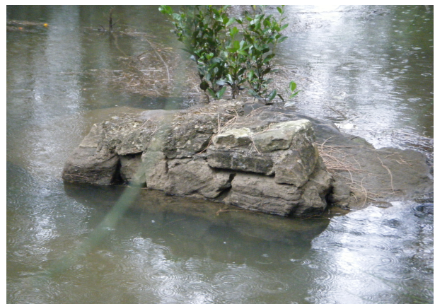
Photo 2: Remains of the ruined older dam – built with old soft cement – probably Lucas'.
