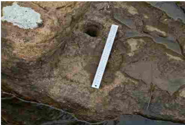
Photo 3: 50mm hole approx 100mm deep. This hole is located in a large, level cut in the bedrock on the river bed, approx 1800mm below cut 1. A large post of 450mm diameter could have stood on this cut and been prevented from moving by an iron bar 'leaded' into the hole (see photo 4). This post probably provided the base for the second of the water wheel's bearings.
