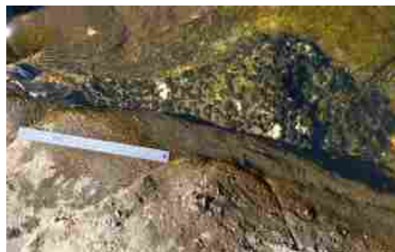
Photo 9: This illustration shows a fissure in the bedrock of the river filled with an estimated 20 litres of cement and basalt aggregate –filling a crack in the river bed in the probable wheel pit. The cement is relatively soft and worn away by water flow.
