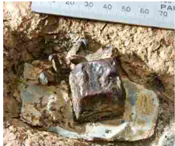
Photo 4: Hole in the bedrock on the river bed. A piece of iron, 25mm x 25mm is inserted into the hole and retained by lead. The iron rod has been broken off at surface level and may be the remains of an iron ring or bar. The hole in the rock appears to be approx 50mm diameter, the same size as holes 1, 3 and 4 which are empty. Also imbedded into the lead are several hand made, steel cut, nails.
