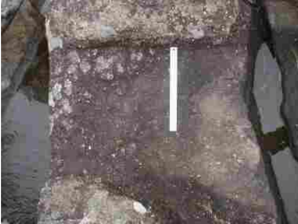
Photo1: Large rock cutting in river bank. This could take a timber beam up to 450mm wide which would have been suitable support for one of the bearings of the water wheel. The wheel pit would be to the left with the river approx 1.5m below the cut.
