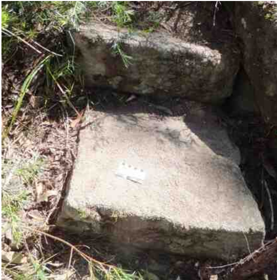
This small section of steps above and west of hut 1 (see map), is made from well-cut dimensioned sandstone. The steps lead towards a Depression-era house site on the dirt road above.
