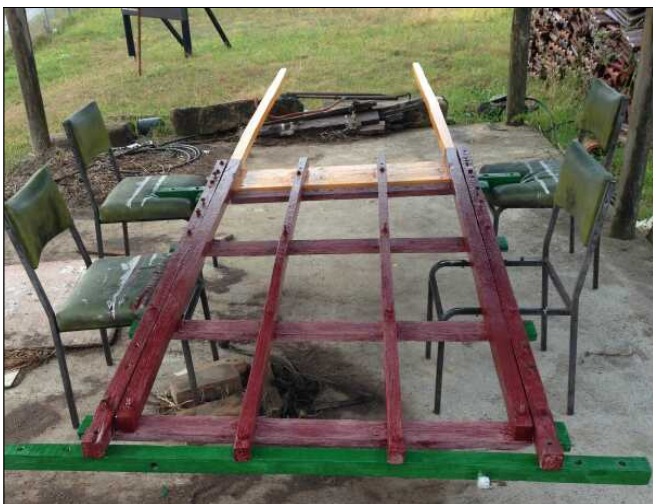
The frame of the cart after it was totally dismantled and one of the wheels in the process of repair.
