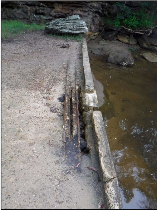
Image 5: Lengths of steel rail from the slipway against the retaining wall [photo G. Jackson]
