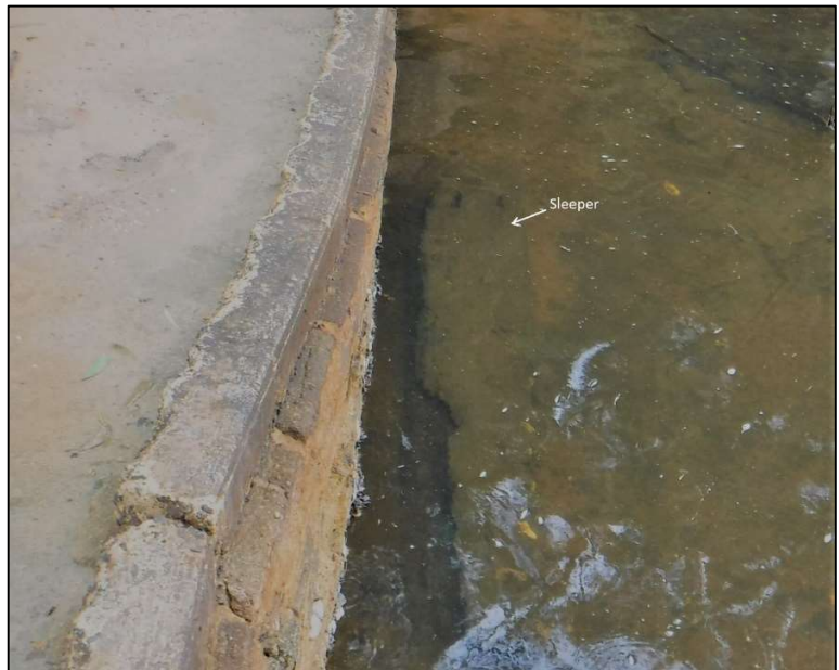
Image 6: Remains of a wooden sleeper visible at low tide beside the retaining wall (this photo has been filtered to improve the visibility of the sleeper) [Photo G. Jackson]
