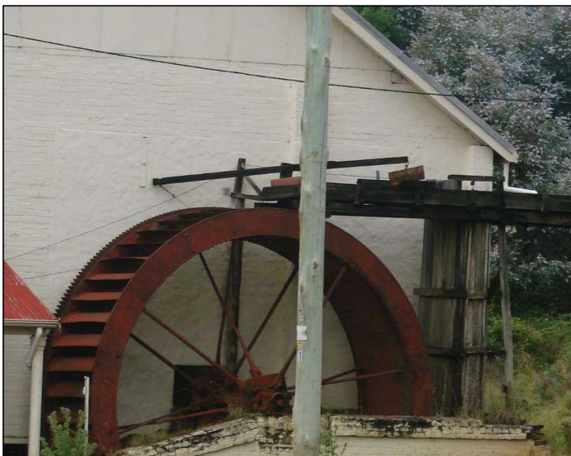
Image 5: This photograph shows a privately owned, un-named rim drive mill near Hobart, Tasmania. The toothed gearing around the wheel's perimeter drives a small cog (not visible) transferring power to the mill's machinery. [Photo by authors, 5 November 2011]
