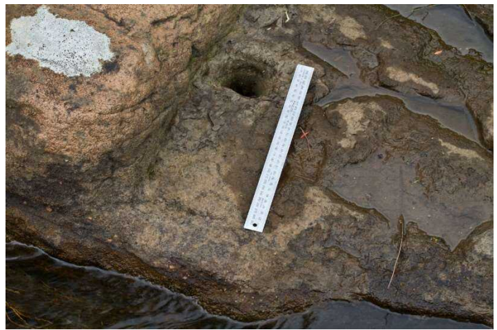
Photograph 4: shows a hole cut in the bedrock on the river bed. A piece of iron, 25mm x 25mm is inserted into the hole and retained by lead. The iron rod has been broken off at ground level and may be the remains of an iron ring or bar. The hole in the rock is approx 50 mm diameter, the same size as hole 1, 3 and 4 which are empty. Also inserted into the lead are several hand- made steel cut nails.
